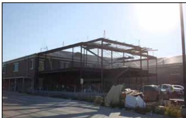
Structural Steel Erection
