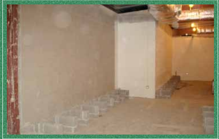
Visitors' Locker Room
