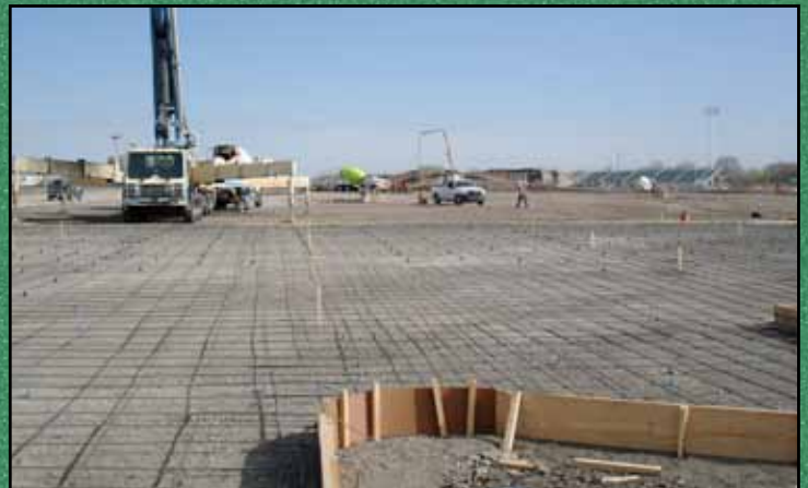
Ninth Grade Center Parking Lot
