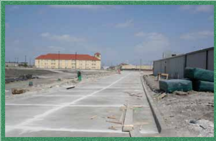
Fire Lane at North End
