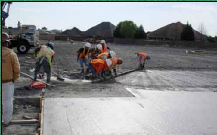
Ninth Grade Center Parking Lot
