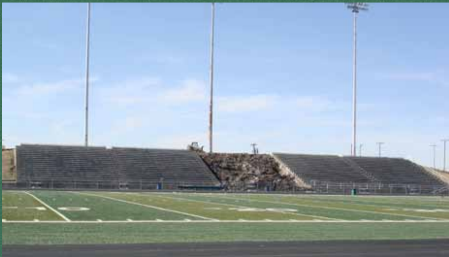
View from field after the press box demolition.
