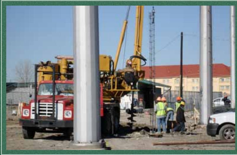
Drilling Piers at Visitor's Side
