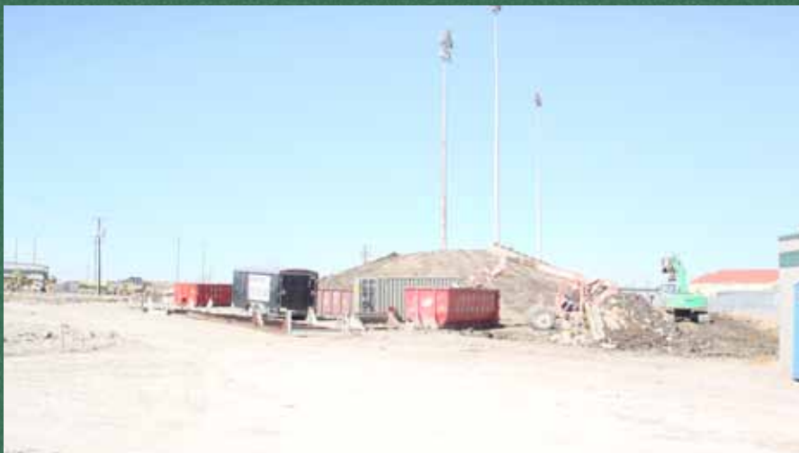
View from parking lot after the press box demolition.
