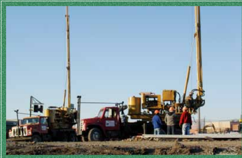
Pier Drilling - Retaining Wall at Visitor's Side
